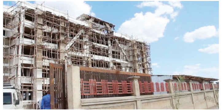
Tanzanite Exchange Centre building almost ready.
